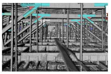
New roof trusses designed by Courts Engineering for Alexandra Palace. When inspecting the roof, Courts noticed targets on the walls indicating that scans had already been done; nobody else had been able to use the data.
