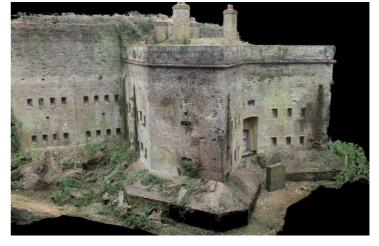
Part of OmegaGeo's point cloud of Leeds Castle, captured using a mixture of terrestrial, aerial and water-based scans. The point cloud was animated using Veesus Arena4D's high-definition point cloud animation functionality.
